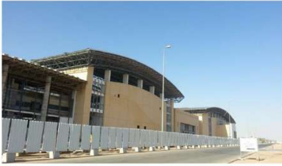
QASSIM UNIVERSITY - WORK UNDER PROCESS
