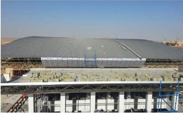
QASSIM UNIVERSITY - WORK UNDER PROCESS
